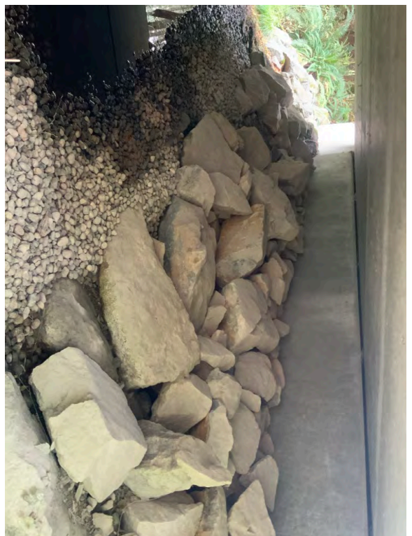
Right Bank Abutment when facing downstream
