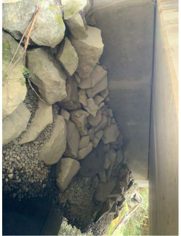
Left Bank Abutment when facing downstream
